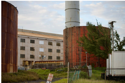
Hawaiian Electric Co.'s Kahului generating station on Maui was commissioned in 1948. (Erin Nolan/Civil Beat/2026)
