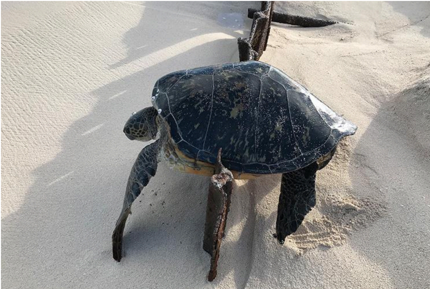
Green sea turtle trapped by decaying infrastructure at Lalo. Credit: NOAA
